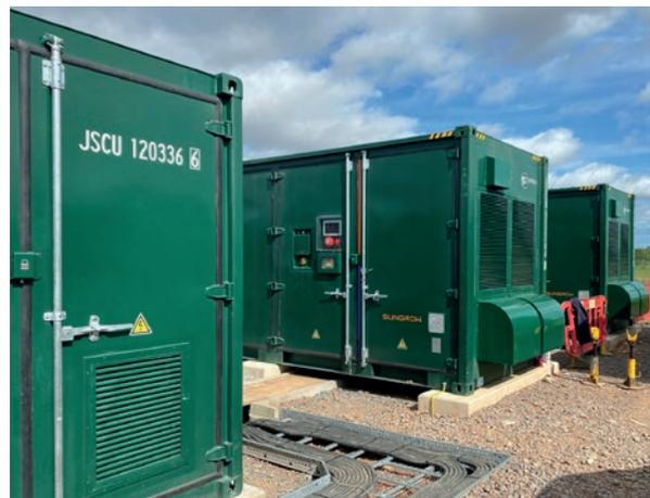
scale up renewable deployment. Helping to balance the variability that comes from natural sources such as wind and solar, the battery is charged when clean energy is abundant and exports it back to the grid during peak times.
