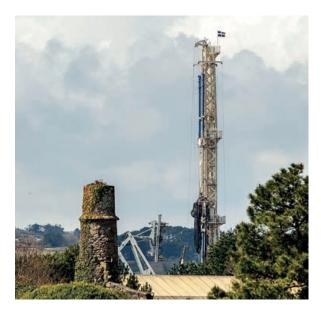
Temperatures in excess of 190°C have been measured in the wells. This natural heat source will be transferred from deep below the surface by water, which will be used to heat a binary power plant. Electricity will be generated 24 hours a day, delivering much needed baseload, which has a crucial role in an increasingly renewables-based grid. The potential for delivering renewable heat locally also begins to address the huge challenge of decarbonising the UK's heat requirement.
