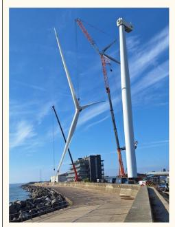
In late 2024, Thrive replaced the nacelle and blades of its Ness Point wind turbine, after nearly 20 years of operation. The replacement turbine parts fitted during the overhaul were refurbished parts from a windfarm in the Netherlands – a great example of reuse which also saves carbon compared to using brand new parts.
